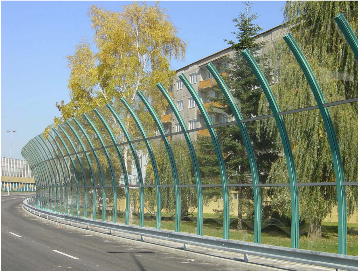
2500 m 2 PLEXIGLAS SOUNDSTOP® XT 15 mm clear Cold bending
