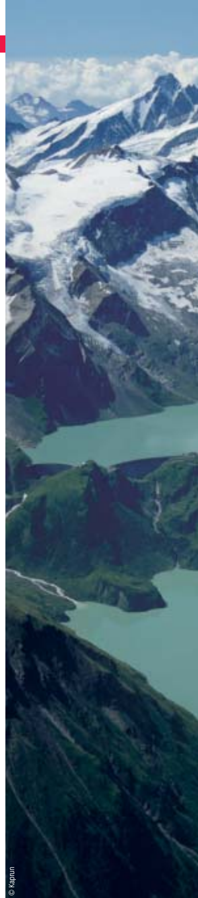
The Verbund is also planning construction of the Limberg 2 pump-fed power station near Kaprun, a project valued at about 365 million euros.
