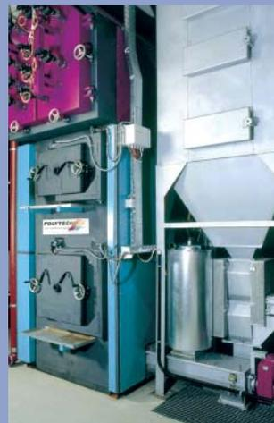
600 kW hydraulic grate firing plant
