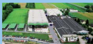
The Posch headquarters in Leibnitz, South Styria.
