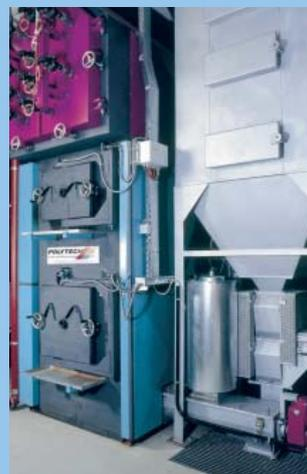
600 kW hydraulic grate firing plant from POLYTECHNIK.
