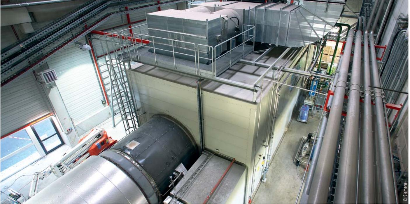
Siemens Power Generation supplied a 40-MW gas turbine and a turbo generator for the paper manufacturer SAPPi's gas- and steam-turbine power station in Gratkorn.
