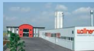
Company buildings ShopCrea wallner. Firmengebäude ShopCrea wallner.
