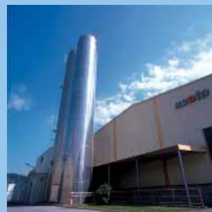
Silos for polypropylene storage with warehouse.
