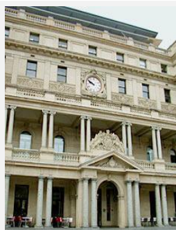
Barnet Long Room Customs House Level 1, 31 Alfred Street Sydney NSW 2000
