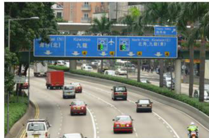
Journey Time Indicators at Gloucester Road Eastbound near Revenue Tower
