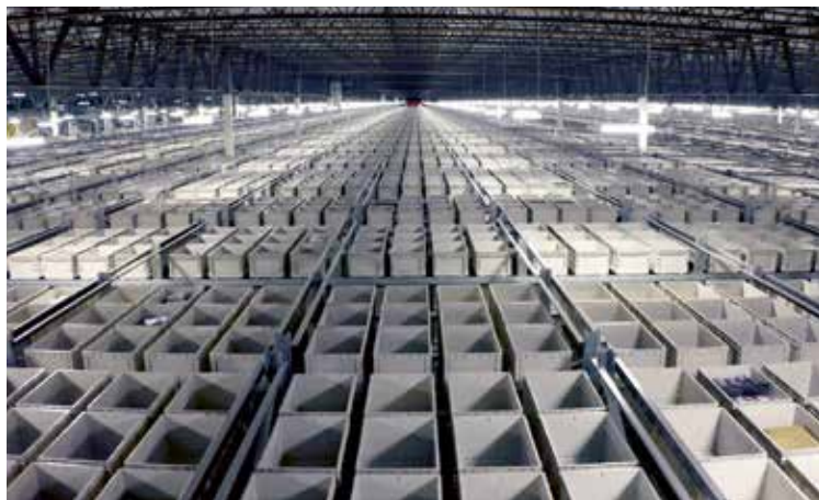
可拓展的科纳普自动存取系统设计 Scalable KNAPP automated storage and retrieval system design
