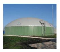
Tank-mounted gas storage installations (pressurised or supported by a mast) are used to store biogas directly on steel or concrete tanks.
