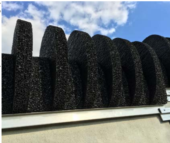
Detail of PIN Lärmspoiler © by CALMA-TEC in Hungary
