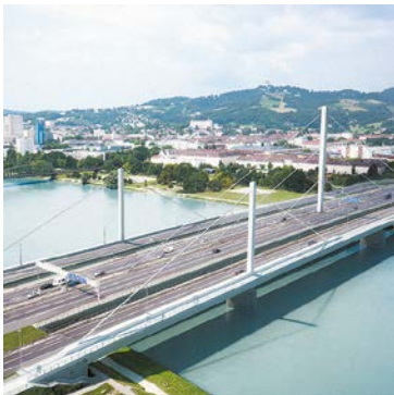
A7 VOEST Bridge, Upper Austria, Austria
