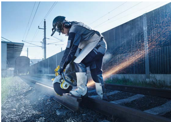
Rail cutting with TYROLIT cut-off wheel
