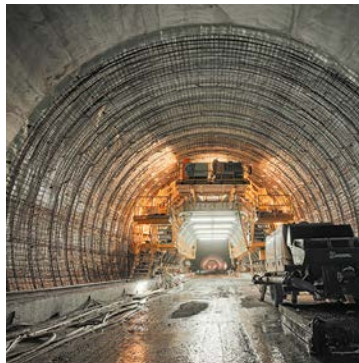
A12 Perjen Tunnel, Tyrol, Austria
