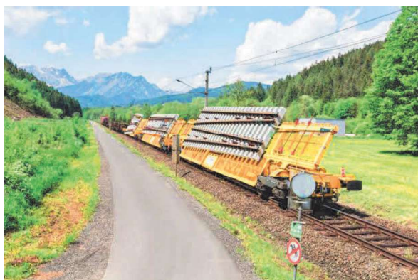
© VOESTALPINE TURNOUT TECHNOLOGY ZELTWEG GMBH
