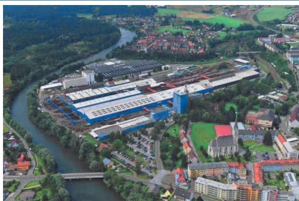
© VOESTALPINE TURNOUT TECHNOLOGY ZELTWEG GMBH
