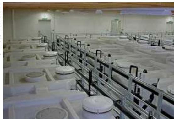
PVS VOPROM WWTP
