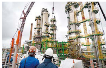
Column replacement in a crude oil plant, Germany
