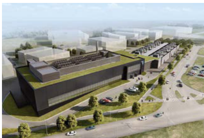
AVL turnkey solutions – early project stage
