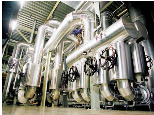
Chemical pipe installation © Foto: SMB
