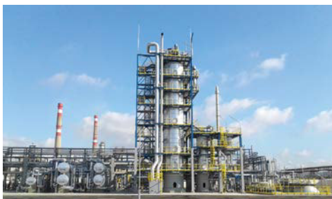
Biturox® plant in Baku, Azerbaijan all pictures © Pörner Ingenieurgesellschaft mbH
