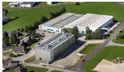
New production building opened in 2020
