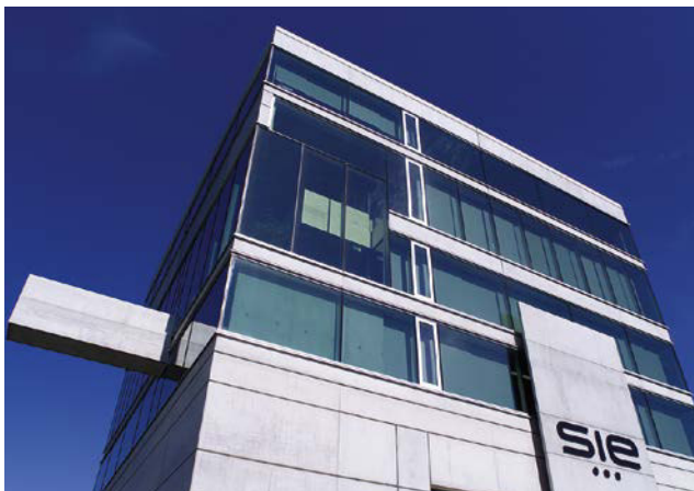
S.I.E Headquarters Lustenau all pictures © S.I.E SOLUTIONS
