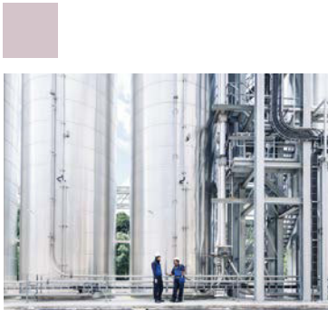
GAW technologies plant construction all pictures © GAW technologies GmbH
