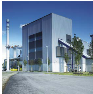
BERTSCHenergy biomass power plant all pictures © BERTSCHenergy GmbH & Co KG
