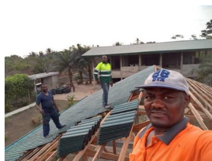
AMABO roof tiles during installation
