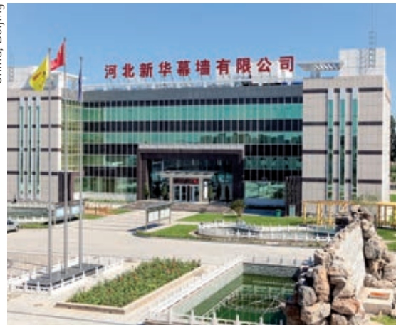
First office building in Passive House Standard China, Beijing
