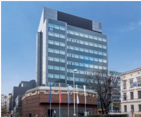
First energy-plus office tower in the World Austria, Vienna
