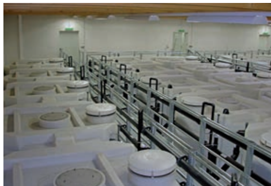
PVS VOPROM WWTP
