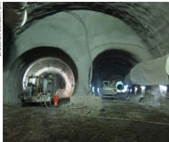
Ready to Spray, Whitechapel Station, Crossrail London, UK
