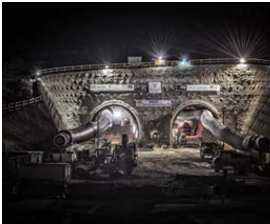
Albasting Tunnel, Wendlingen – Ulm, Railway, DE
