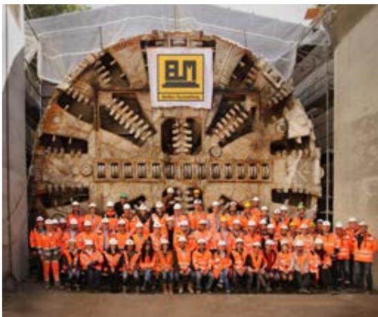
Slurry TBM with BeMo team, Metro Karlsruhe, Germany
