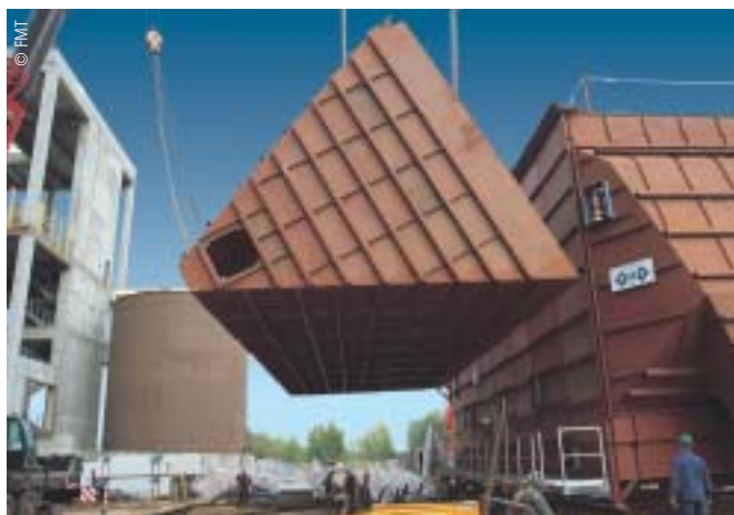
FMT assembly work at the Stendal cellulose woodpulp works.
