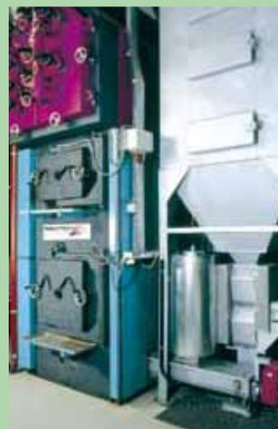
600 kW hydraulic grate firing plant
