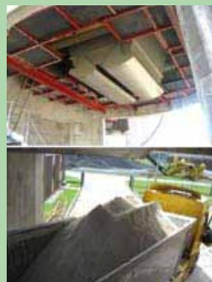
Removal of 12% moisturized FGD gypsum from a concrete silo 600m<sup>3</sup>, diam. 8m.
