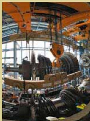
Installation of turbines in a combined cycle power plant.
