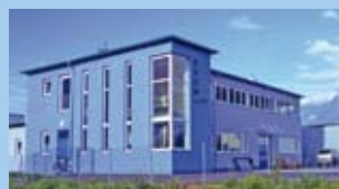
Production building in Mils, Tyrol.
