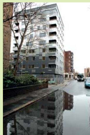
Murray Grove - tallest timber residential building in the world. Murray Grove – höchstes Massivholzhaus der Welt.
