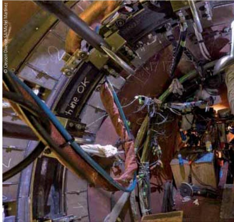
A prestigious project completed by MCE AG: the replacement of the pressure shaft cladding at the Cleuson-Dixence hydropower station in the Swiss canton of Wallis.
