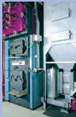
600 kW hydraulic grate firing plant
