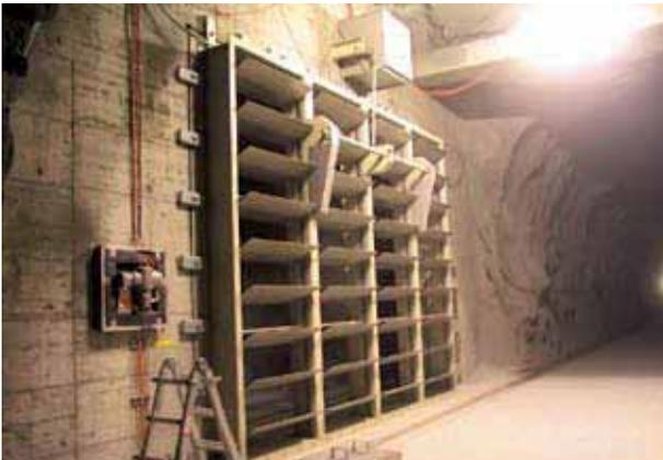
Ventilation / smoke extraction / controll dampers for tunnel systems • Special fans for the process industry (power stations, cement plant etc.)
